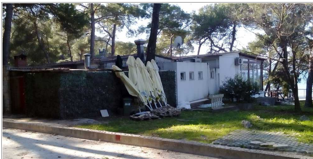
Gradevina 1 – pogled istok
